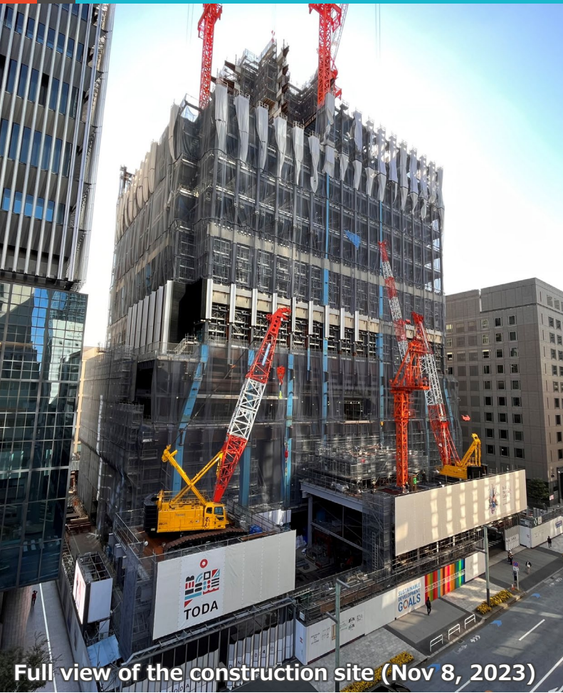
System scaffold climbing status (core wall 15F)
