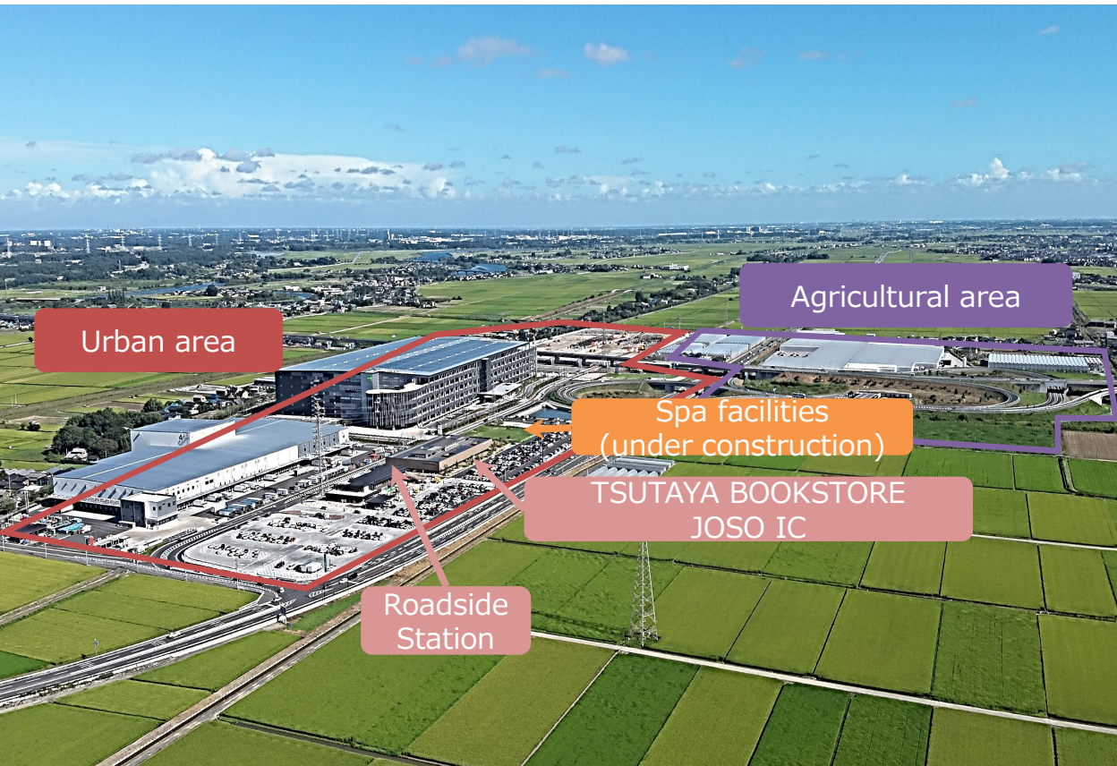
Panoramic view of Joso Project
