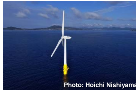
Floating offshore wind turbine generator
