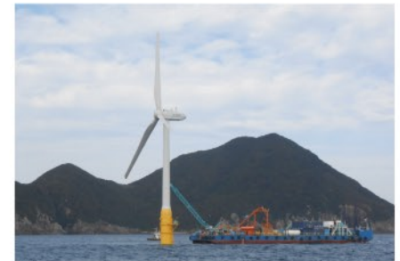
6. To complete the installation, mooring chains and submarine cables are connected to the turbine at the installation site.
