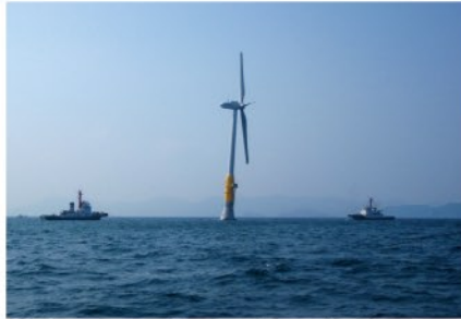
5. After its completion, the wind turbine is towed from the assembly site in the sea north of Kabashima to the installation site.
