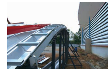
Field test of eaves (truck berth portions) with curved shape.
