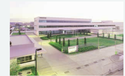
Bridgestone Asia Pacific Technical Center Co., Ltd. New Research Center BRIDGESTONE ASIA PACIFIC TECHNICAL CENTER CO., LTD.
