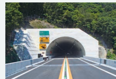
Kinki Regional Development Bureau, Kisei Line Wabukagawa Tunnel construction Kinki Regional Development Bureau, Ministry of Land, Infrastructure, Transport and Tourism
